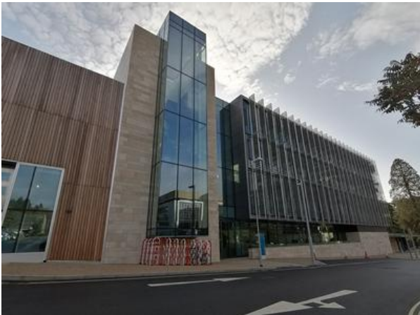
National Infrastructure Laboratory at Boldrewood
