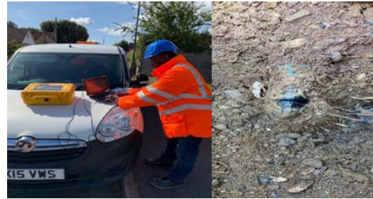
Figure 1. Leak detection & excavation
