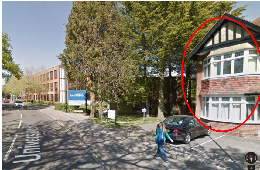
Street View of the Wellbeing Centre
