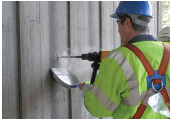
Use of percussive or rotary action tools may put users at risk of vibration injury
